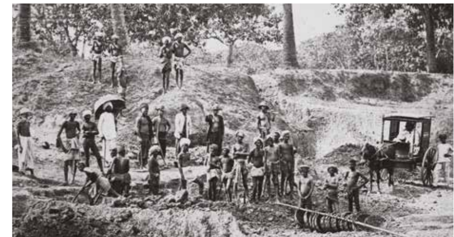
The British East India Company brought prisoners from India to Singapore to build the settlement's early infrastructure. One of the prisoners' early tasks included transporting soil from Pearl's Hill and Bras Basah as landfill for the marshy area that would become the commercial hub of Singapore. Courtesy of National Museum of Singapore, National Heritage Board.
